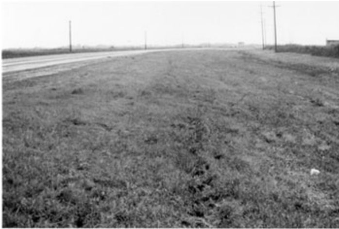
Exhibit 3-53: Typical roadway with Roadside Hazard Rating of 2
