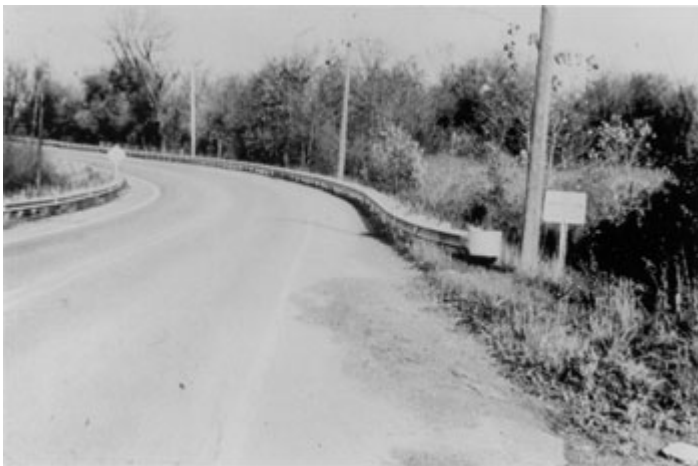
Exhibit 3-55: Typical roadway with Roadside Hazard Rating of 4
