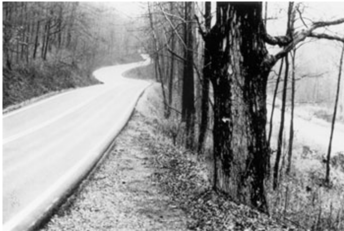
Exhibit 3-57: Typical roadway with Roadside Hazard Rating of 6
