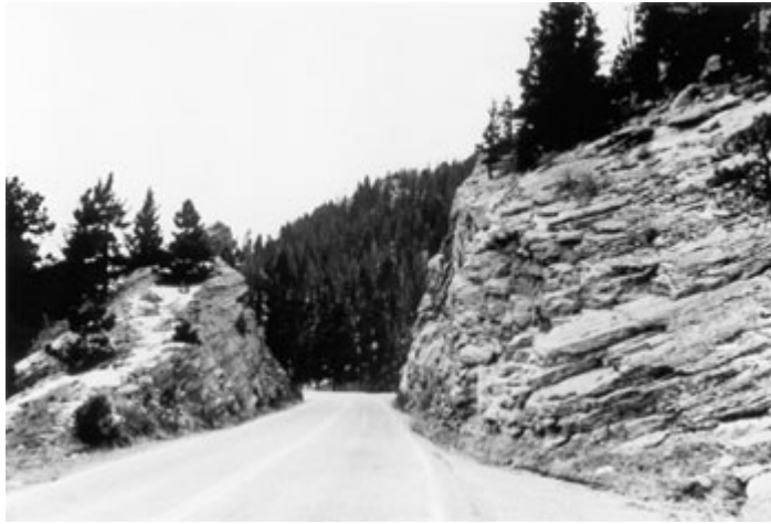
Exhibit 3-58: Typical roadway with Roadside Hazard Rating of 7
