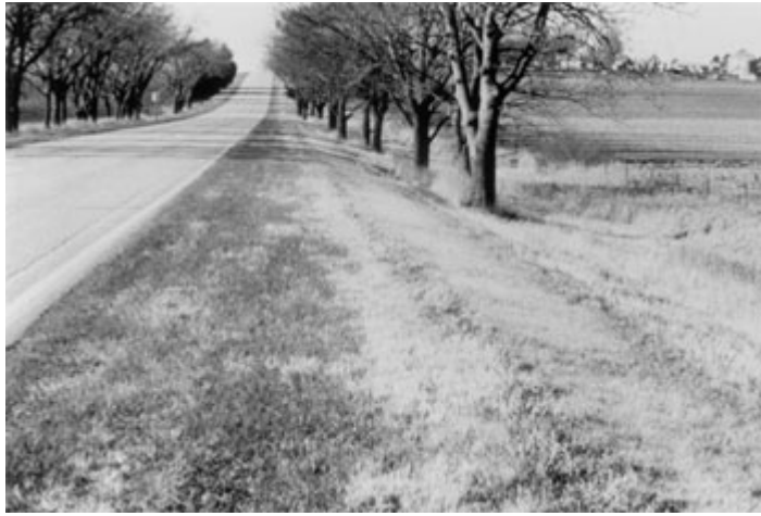
Exhibit 3-56: Typical roadway with Roadside Hazard Rating of 5
