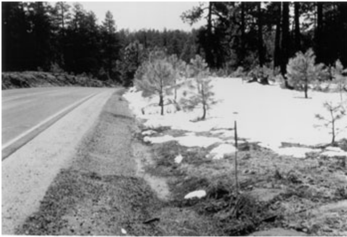
Exhibit 3-54: Typical roadway with Roadside Hazard Rating of 3
