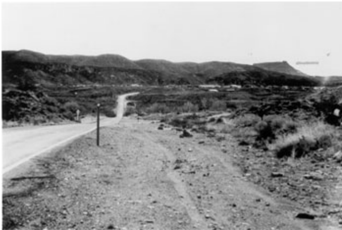
Exhibit 3-53: Typical roadway with Roadside Hazard Rating of 2
