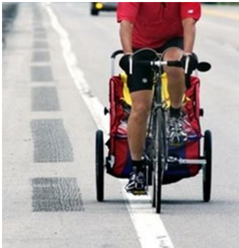
Figure 2.2 Intermittent Rumble Strips on 3 ft. Shoulders
