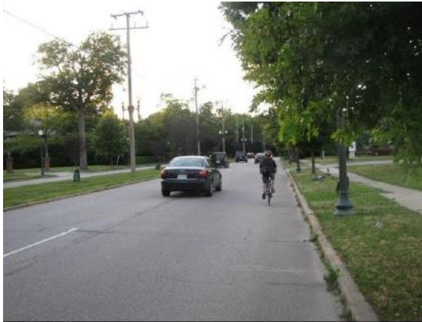
Figure 2-7: Wide Curb Lane (Source: Mead et al., 2014) (Photo Courtesy: James and Gilbert, 2012)
