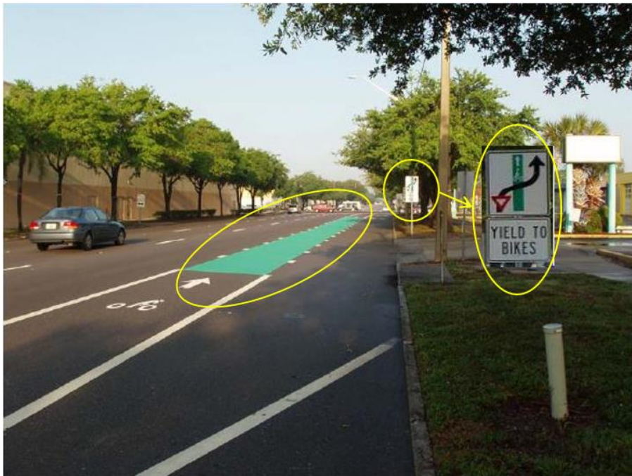
Figure 2-4: Green-colored Pavement and Accompanying Signing in a Bicycle Lane Weaving Area in St. Petersburg, FL (Source: Hunter et al., 2008)
